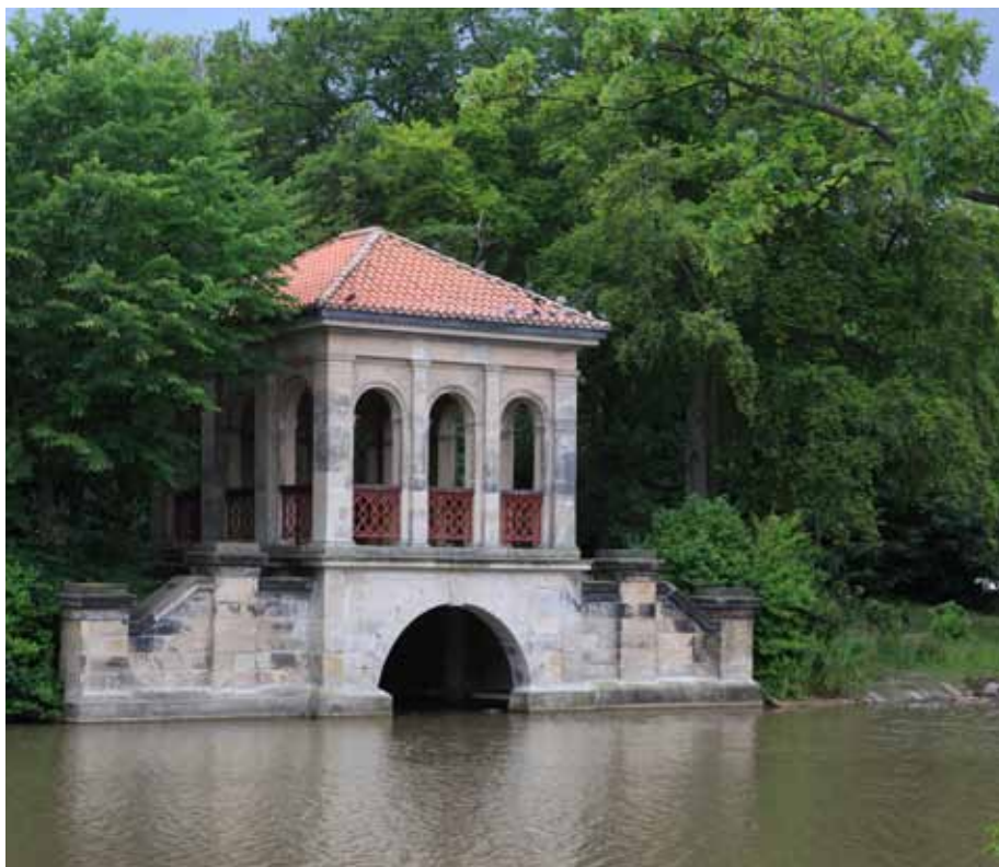
Restored Roman Boathouse - Paxton's idea for a Bandstand
